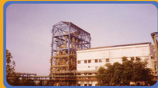
Fumaric Acid and Malic Acid Plants under Construction in 1996.
