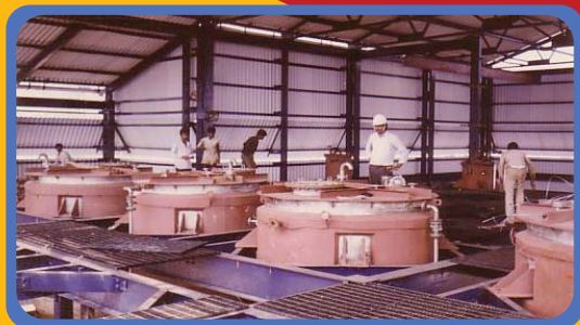
Construction of the Malic Plant – March, 1992 .
