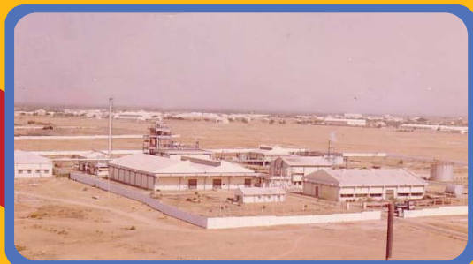
The TCL's first PA Plant in Ranipet, March 1976 .
