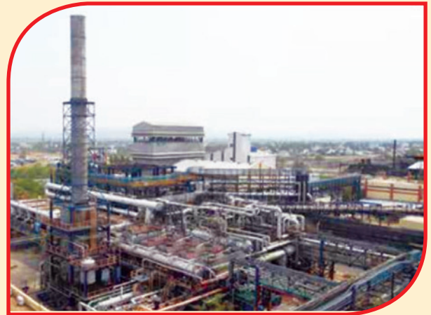
PA Plant - Ranipet, during revamp
