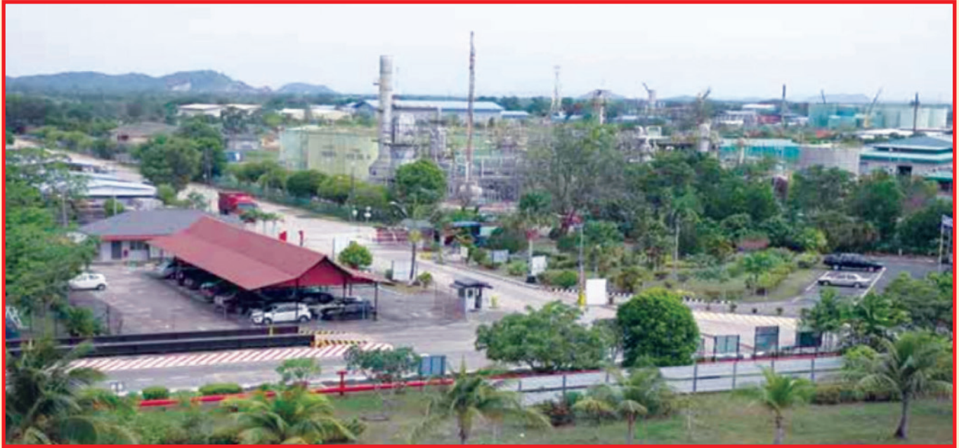
Overview of our subsidiary in Malaysia - The Maleic anhydride Plant
