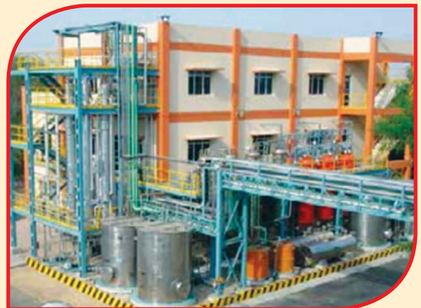
A section of the Fine Chemicals Plant
